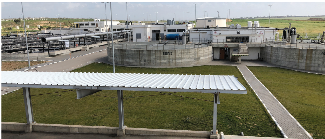
Picture from UNEP visit to the North Gaza Emergency Sewage Treatment plant (NGEST). Solar covers half of the plant's energy operation requirements. Re-charged water will be sent to the aquifer and then will be used for irrigation. Plans exist for bio-gas production in the future. (Ron Witt)
