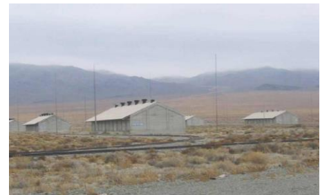
Fig. 10: Warehouses used for above-ground storage of elemental mercury
