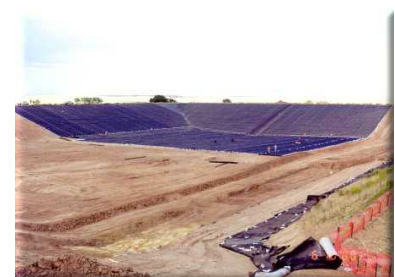
Fig. 12:A specially engineered landfill
