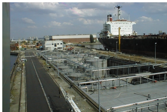
Fixed PRF in port of Antwerp (Belgium) (Photo credits: MAC 2 )
