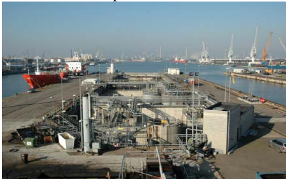
Fixed reception and treatment facility (Photo credits: MAC 2 Antwerp, Belgium)
