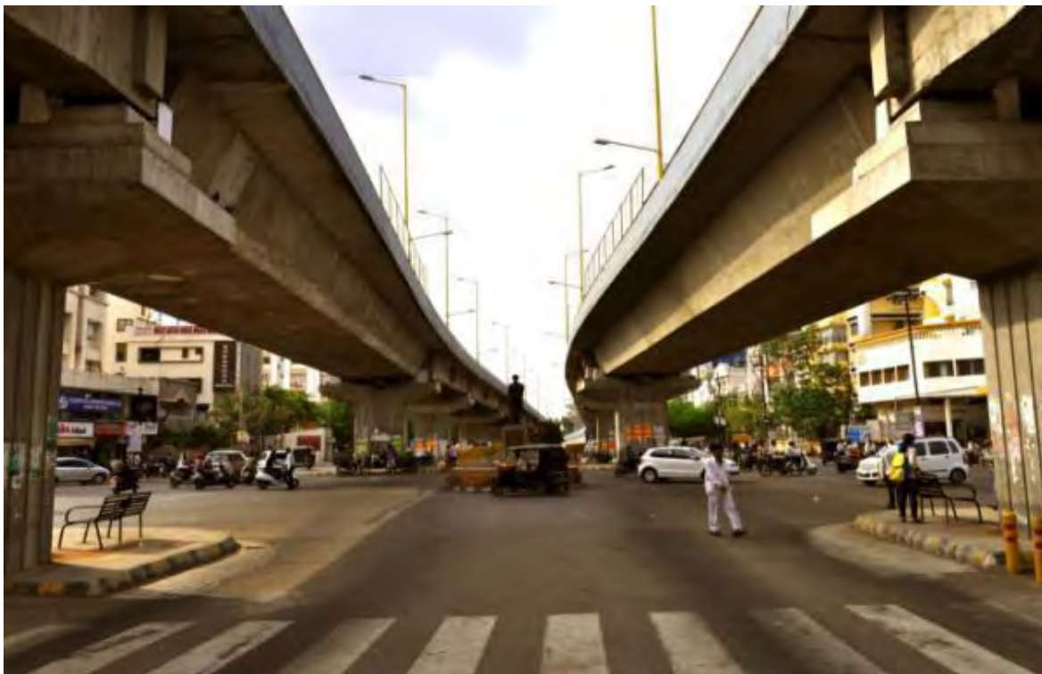
Figure 3-16: Image showing flyover at KKV Circle
