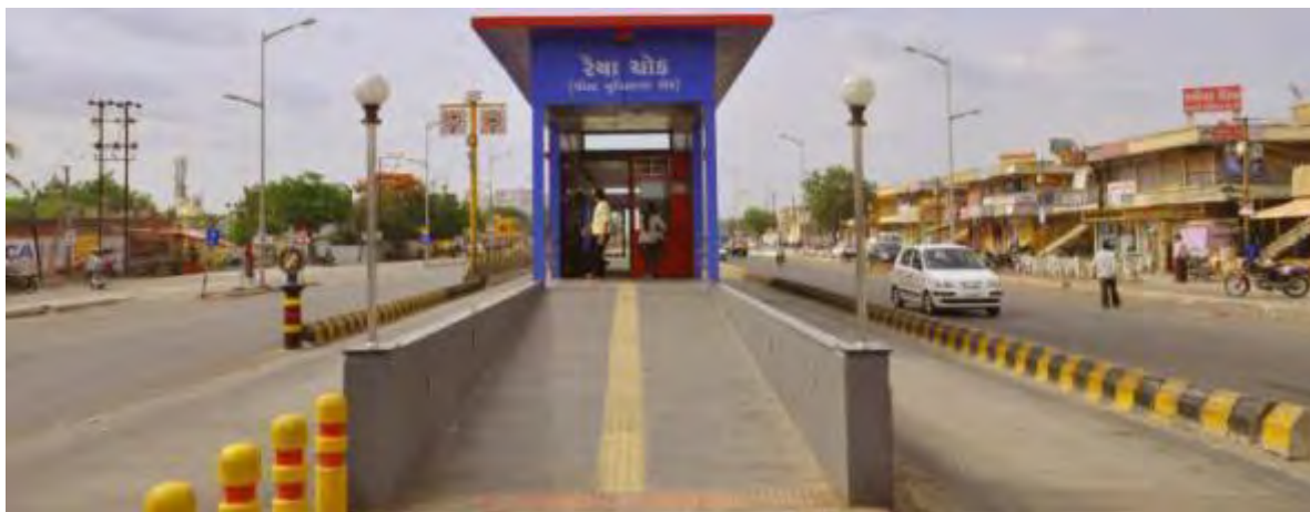
Figure 3-9: BRTS stop at Raiya Chowk
