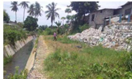
*The Ilala drainage canal prevents floods that used to reach adjacent dwellings (reinforced with barriers of loose stone and rubble).*
