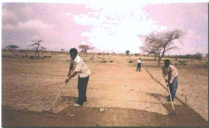
Clearing ground for school construction
