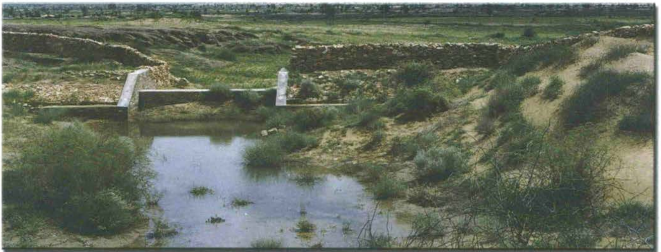
Community water-harvesting through water dam construction
