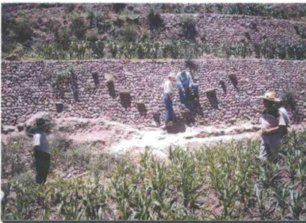
Rehabilitation of terraces on hillsides
