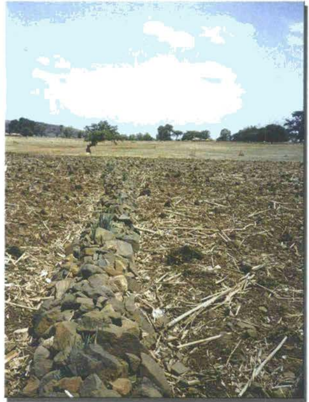
Vegetation and stones are used to build anti-erosion dykes
