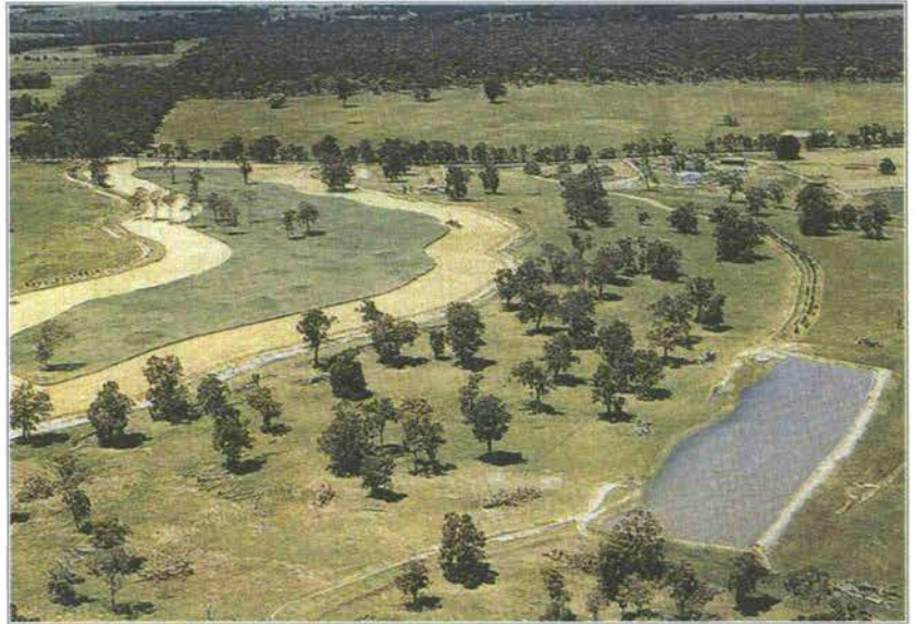
A contour check dam stores water for irrigation
