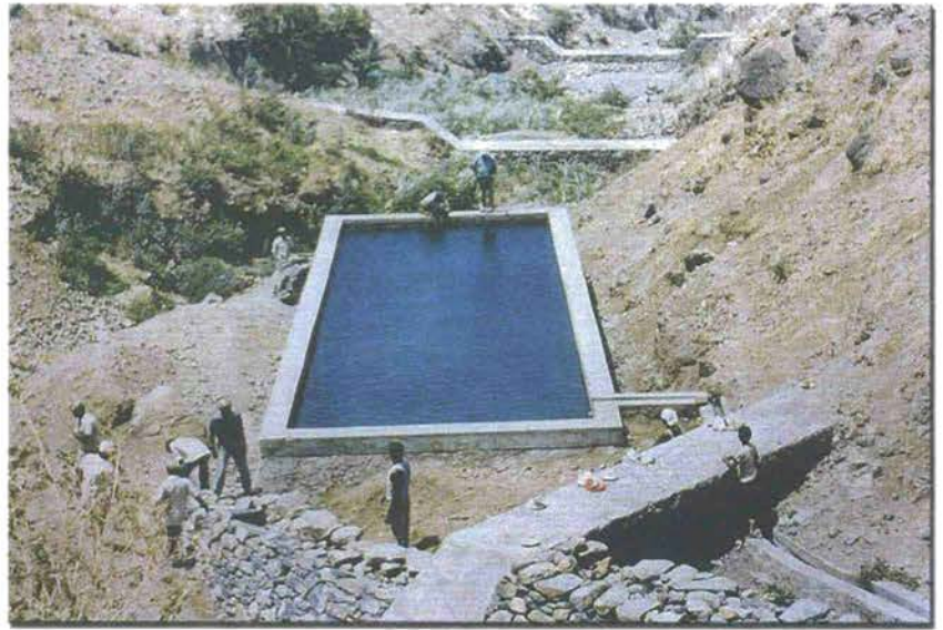
Construction of a catchment channel, reservoir and erosion control masonry
