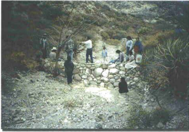
Building stonework systems to harness water and control soil erosion
