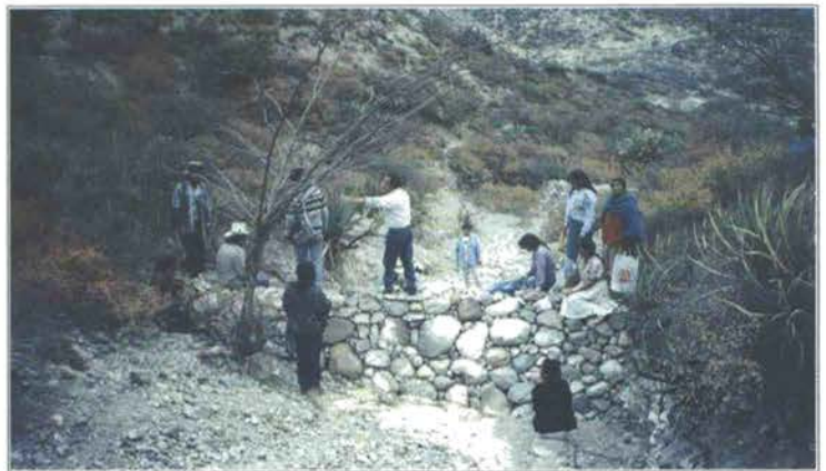
Building stonework systems to harness water
