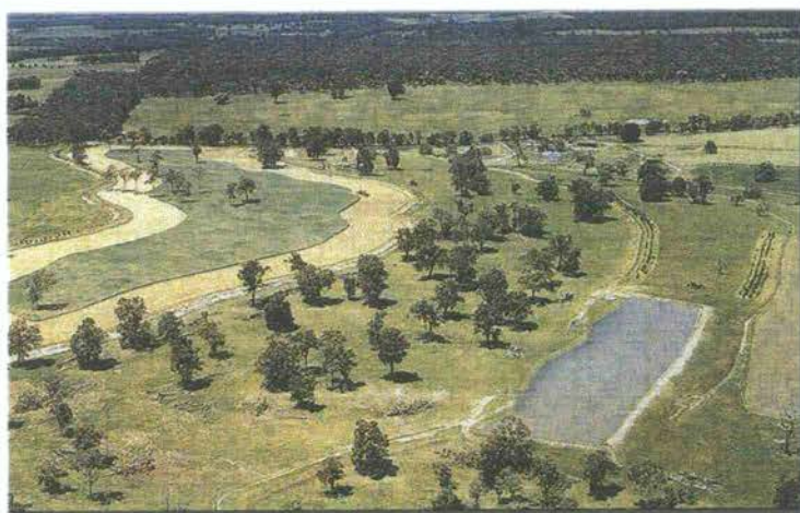
A contour check dam stores water for irrigation
