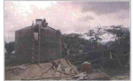
Constructing a water storage tank
