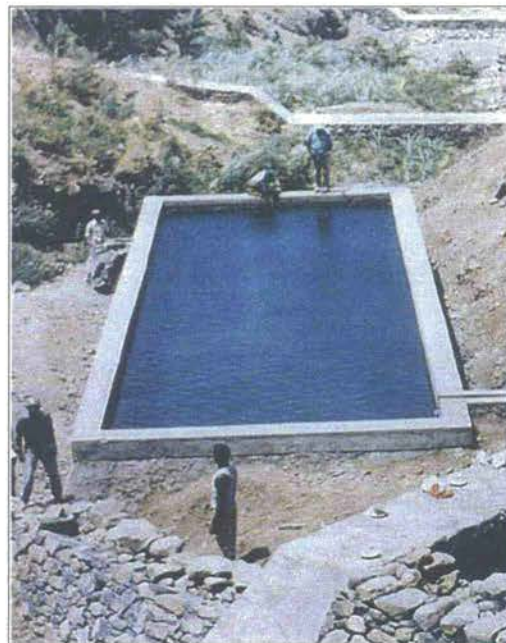
Construction of a catchment channel, reservoir and erosion control masonry
