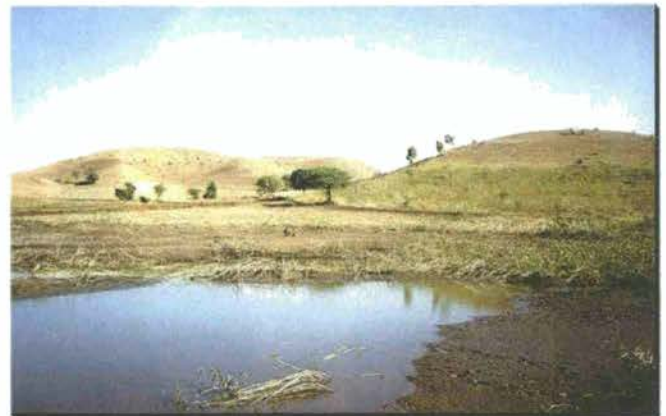
Community water-collecting dam
