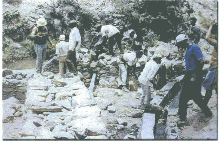
Community members build an irrigation channel
