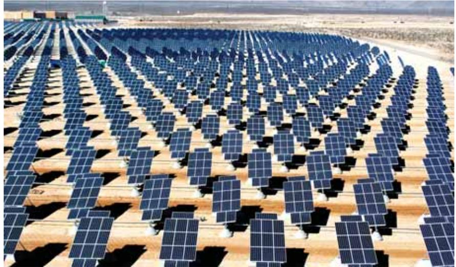
These 70,000 solar panels were placed on 140 acres of unused land, and make up just one third of Nellis Air Force Base, Nevada's solar arrays, the largest photovoltaic system in the Americas. Base officials and SunPower Corp. finalized a commission of 14.2 megawatts in solar power that is reported to save Nellis AFB \$1 million annually and provide about 25% of the base's electricity requirements.
