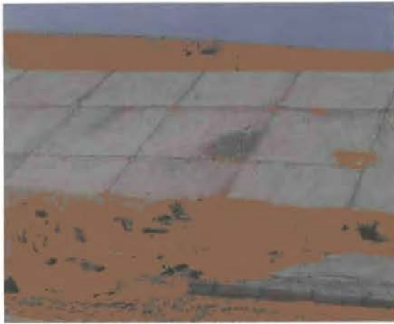
Sand traps for sand dune fixation.
