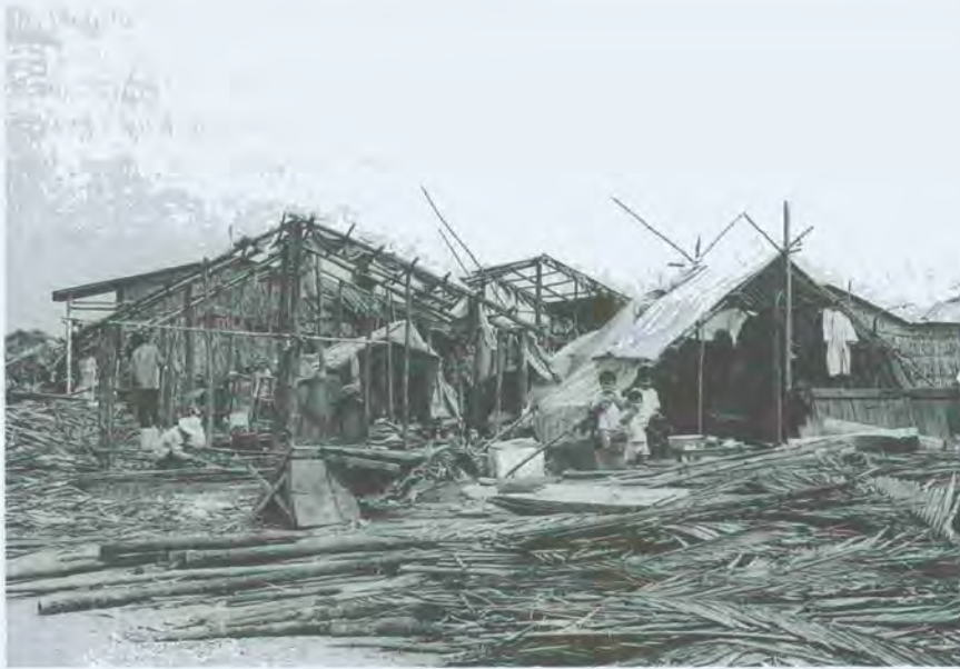
Fig. 5 El Niño-related storm damage in Vietnam (courtesy N. H. Ninh)
