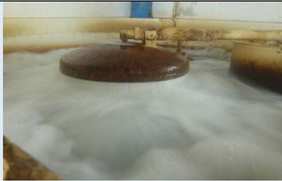
Figure 174: Water pressure dissipation using a load breaker
