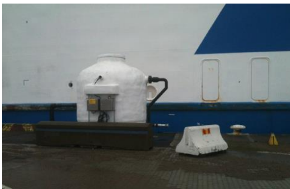
Sewage collection in Trelleborg port (Sweden) (Photo credits: Clean Baltic Sea Shipping)
