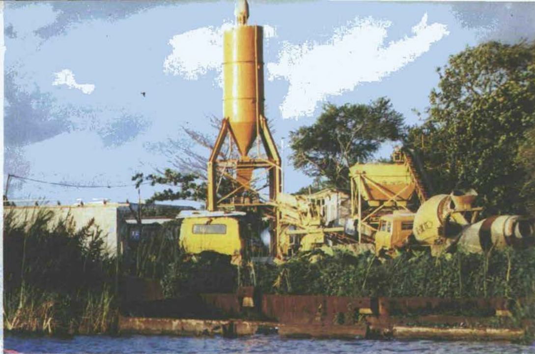
A coastal factory. The Regional Seas Programme has helped Indian Ocean states to develop common environmental standards with regard to effluents which are hazardous to ecosystems and human health.
