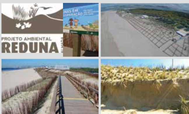
Figure 3.11.2. Dune restoration in Almada, Portugal: signage (A); support structures and native species used to restore the ecosystem (B); overhanging walkways (C); revegetation has withstood recent storms (D)
