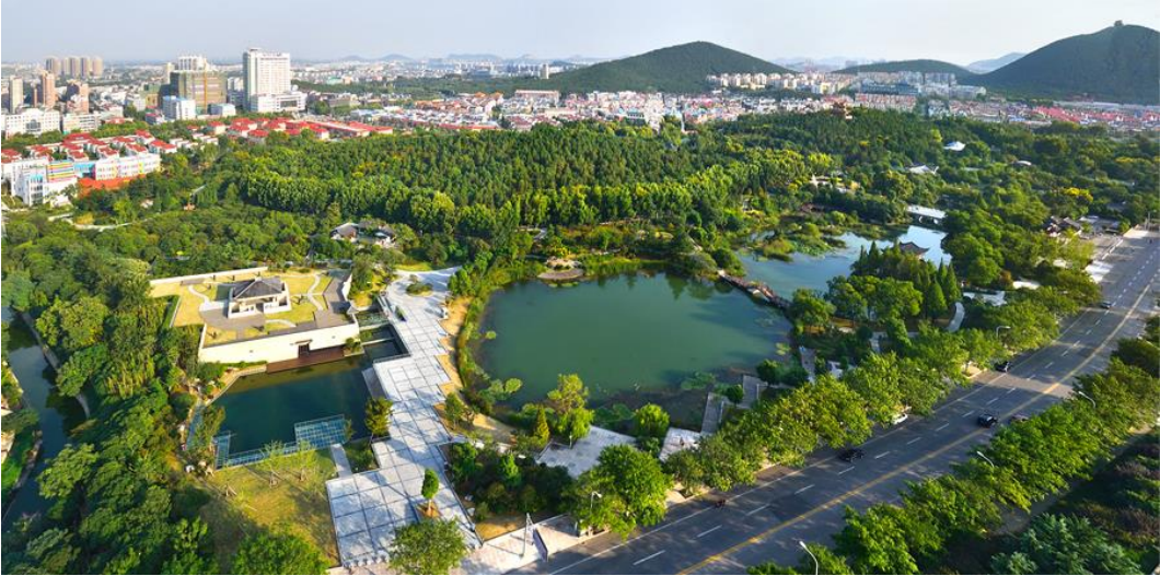
Figure 3 : A panoramic view of Peng Zu Yuan after its renovation in Xuzhou
