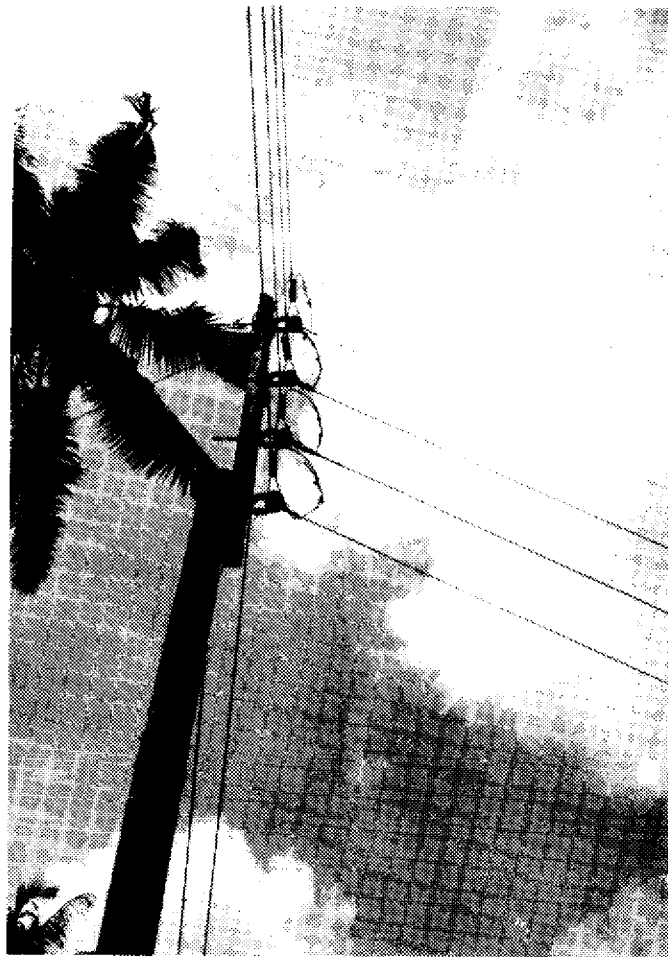
Fig. 11. The Transmission Lines at Dagohoy
