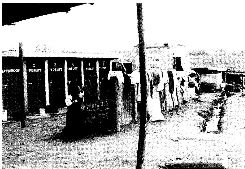
Figure 5.10 Community VIP toilets and water tank in Kibera slums (June 2006)
