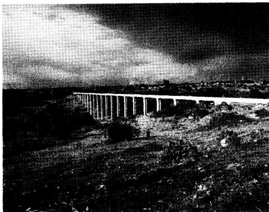
Figure 3.14 Aerial crossing, sewer line 52 – Eldoret Sanitation Project
