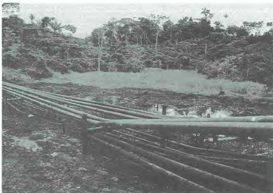
Fig. 33. Pipeline rupture close to well No. 01 in the Aguarico field. The oil flowed into the swampy depression in the background from where the major part was recovered.
