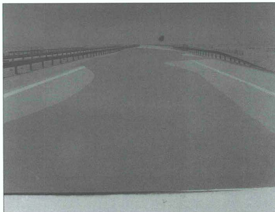
Creeping sands submerge the highway road.
