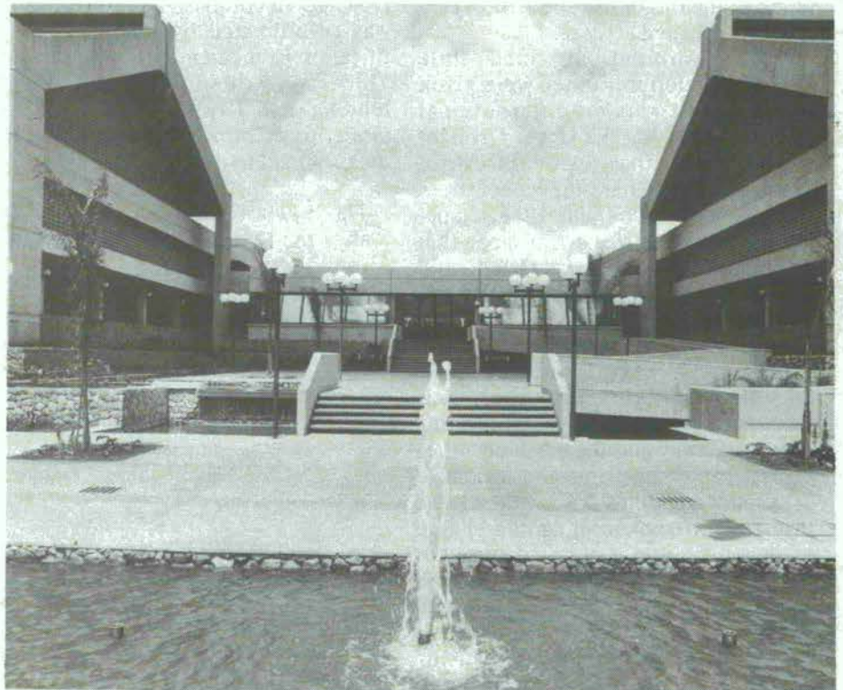
The new United Nations Office complex in Nairobi which was inaugurated at UNEP's twelfth Governing Council in May 1984.
