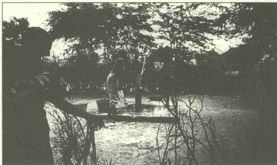
Figure 2.- A water pump at Maho Ly village
