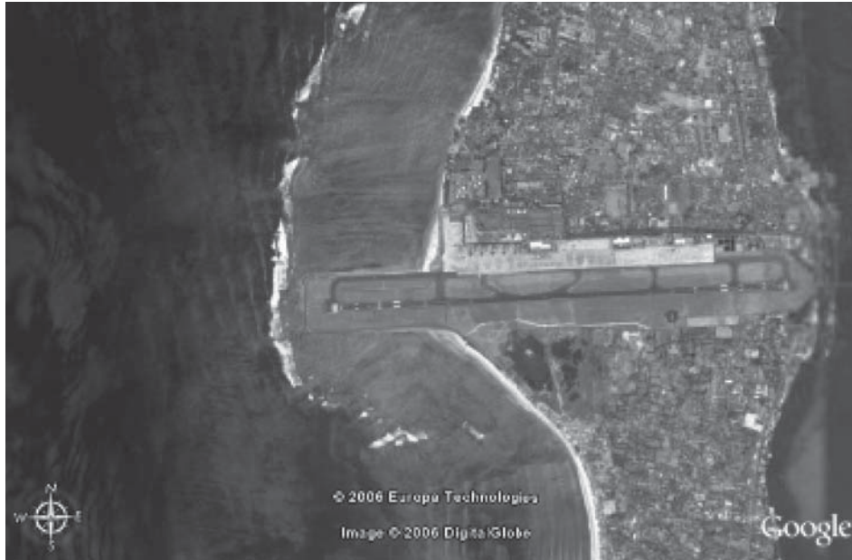
Figure 1.5 Ngurah Rai International Airport Runway Extension that Caused Down-drift Erosion, Kuta Bali, Indonesia
