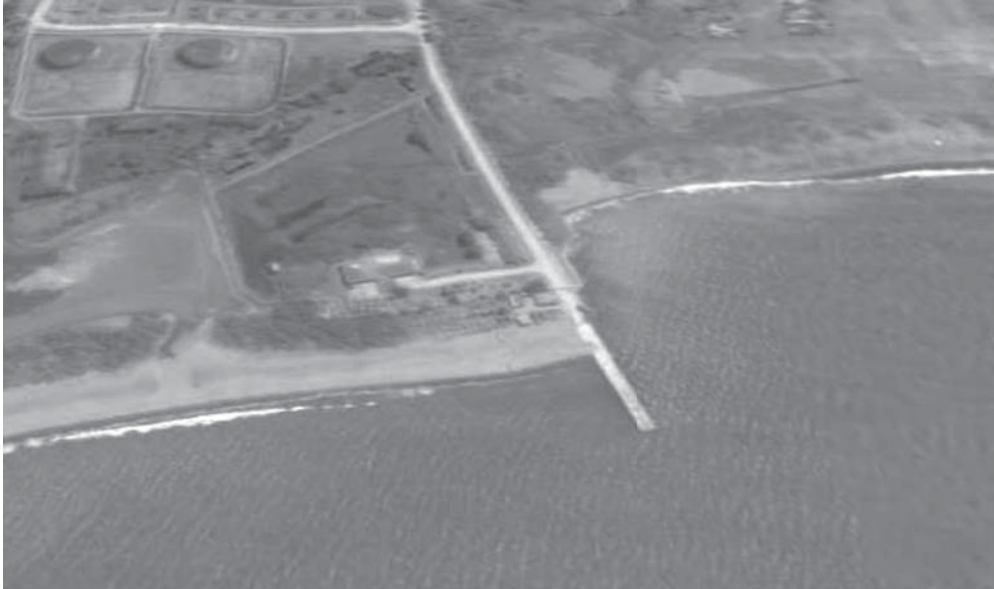
Figure 3.7 Updrift Deposition and Downdrift Erosion at a Jetty, Philippines
