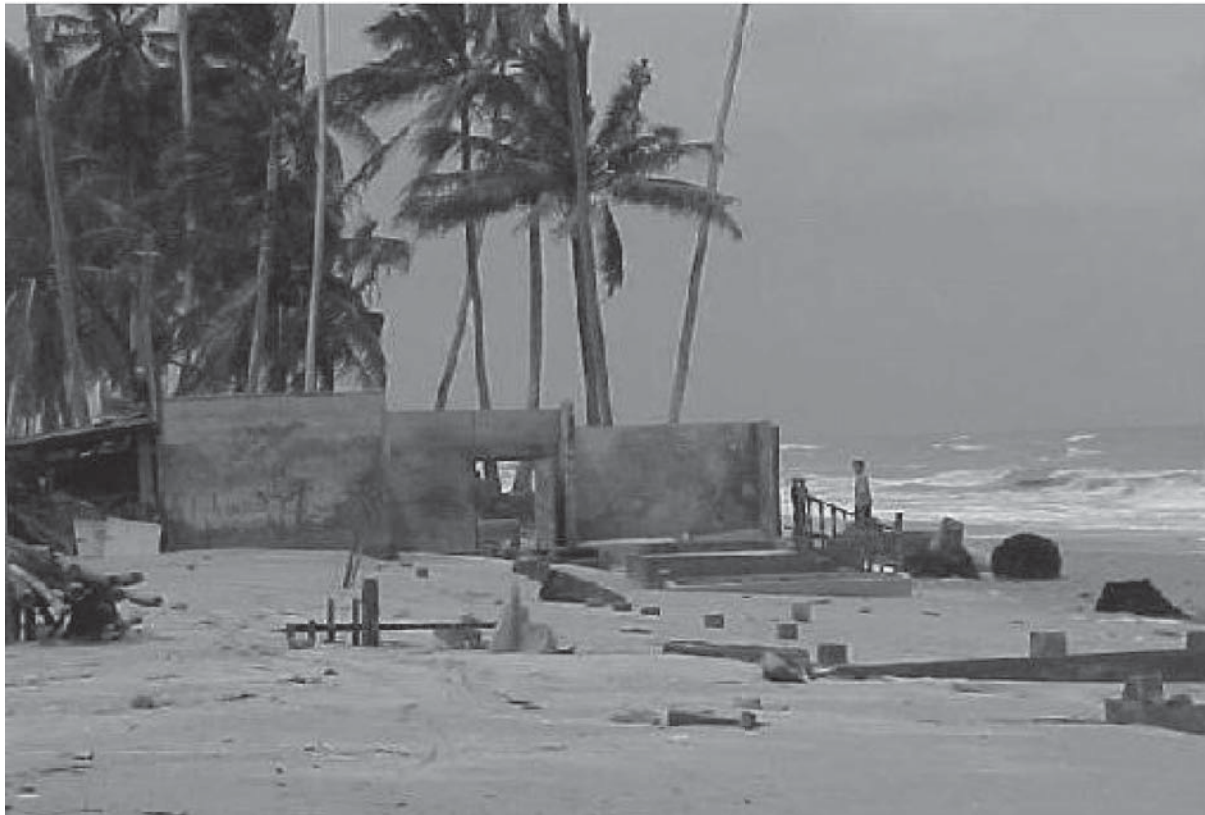
Figure 3.1 Erosion Destroys Coastal Community in Pantai Sabak, Kelantan, Malaysia
