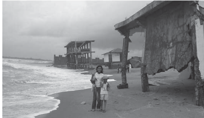
Figure 1.2 Erosion Impacts on the South Bank of the Bucao River Mouth, Botolan, Zambales, Philippines
