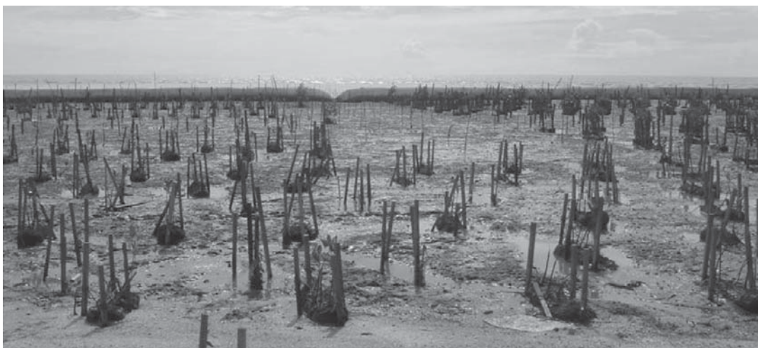
Figure 3.9 Geotube Breakwaters (in background at waterline) and Mangrove Reforestation in Malaysia
