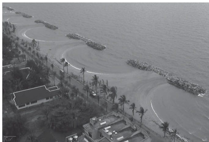
Figure 1.3 Hard Engineering Structures to Mitigate Erosion and Restore Beaches, Thailand
