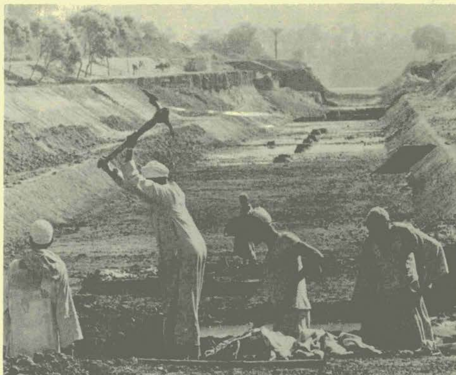
Building a main drainage canal along the banks of the Nile within view of the Valley of the Kings, Egypt. Part of an irrigation system financed by the World Food Programme. Photo: FAO-WFP
