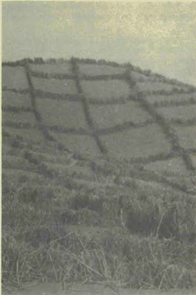
Sand dune fixation experimentation at Repetek Desert Reserve, Turkmen republic, USSR. This is the chessboard method in which sticks 50 cm long are used to mark out the squares. It is said to be a traditional method. Sand accumulates inside the squares.
