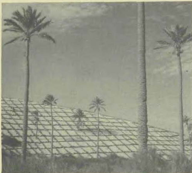
Examples of dune fixation by the "chessboard" method in Libya.
