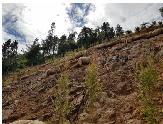
Photograph 1 & 2 – example of terracing using coir logs on a landslip.
