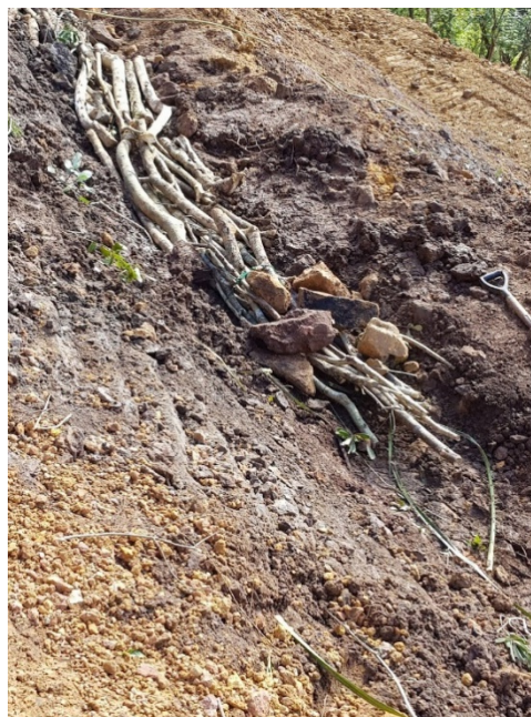
Photograph 3 & 4 – example of fascine drains on a landslide.
