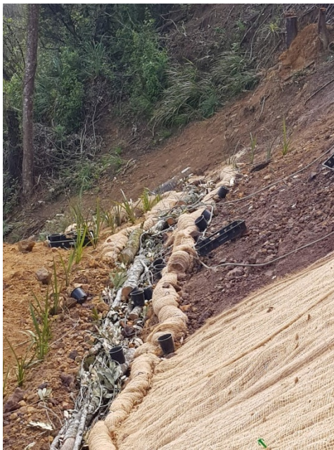
Photograph 3 & 4 – example of fascine drains on a landslide.
