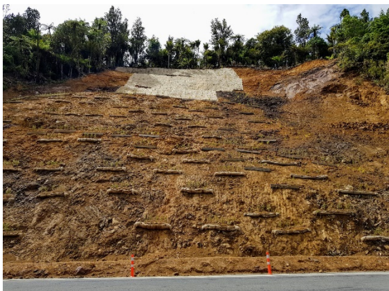
Photograph 1 & 2 – example of terracing using coir logs on a landslip.
