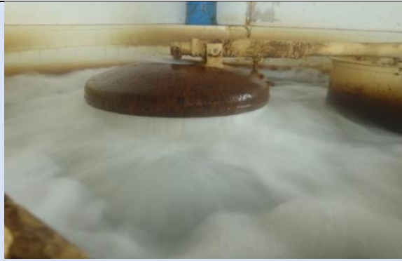
Figure 161 Water pressure dissipation using a load breaker
