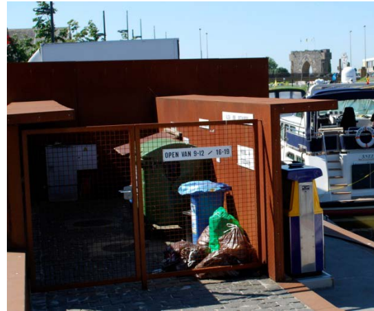
Combined reception facility for bilge water and garbage in a marina in Belgium (Photo credits: Peter Van den dries)
