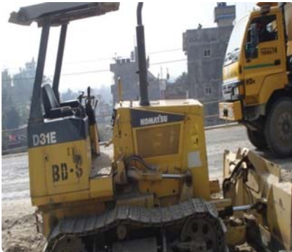
Bulldozer at work
