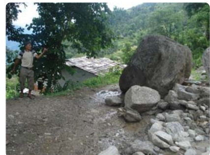
This large stone threatens 36 houses below on the Barabise–Thingsang road
