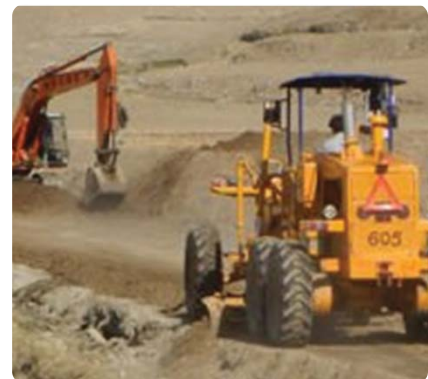
Leveller and excavator at work
