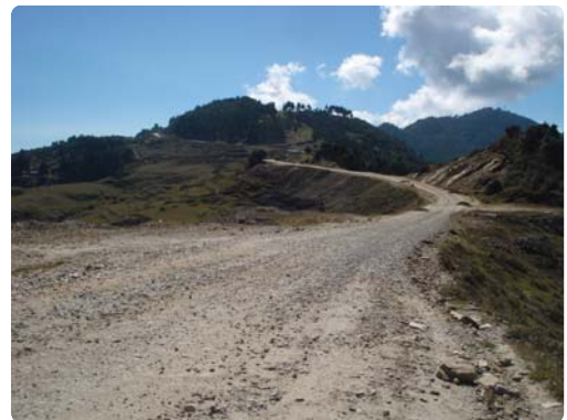
A ridge alignment in Dolakha that may be ideal for EB technology to expedite road construction
