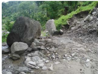
Temporary passage for vehicles opened up without attending to the threat
