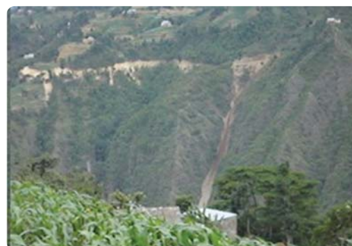
Typical alignment and debris disposal of EB road, Lalitpur district
