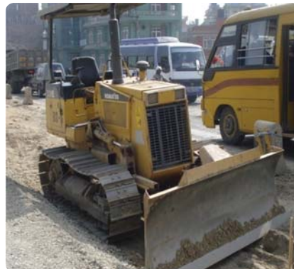
Bulldozer at work
