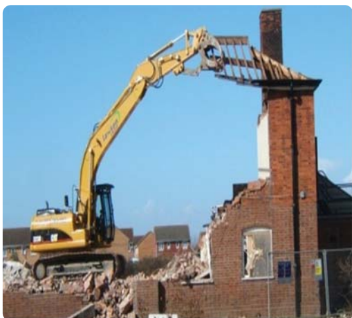
Excavator demolishing a house
