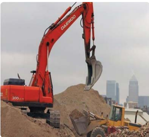
Excavator at work
