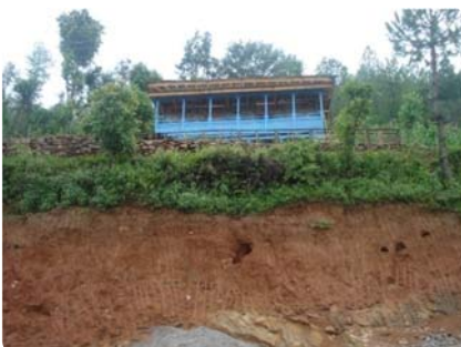
Former house of Sitaram Bishwakarma along Bhirkot–Chhaunde road
