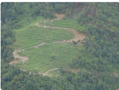
Typical new alignment feature of an unplanned VDC road in Sindhupalchok
