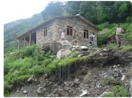
Community building endangered by landslide
