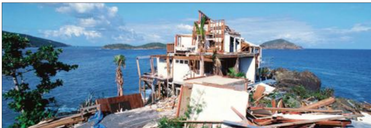
Destruction after hurricane
