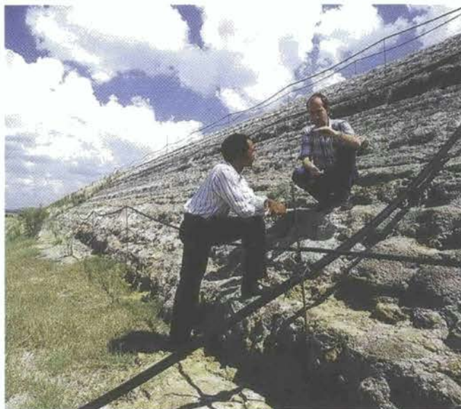
Monitoring successful tailings dam vegetation program.
