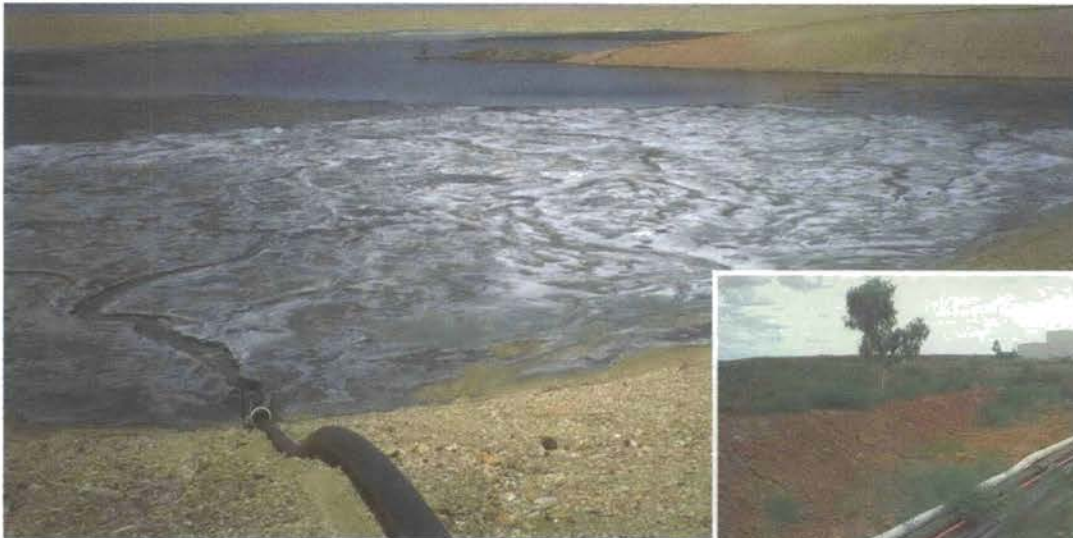
Tailings delivery and return lines are located in an earth bund containment system which will hold a full line rupture from any line for a minimum of four hours. The lines are inspected physically every four hours for leaks.
