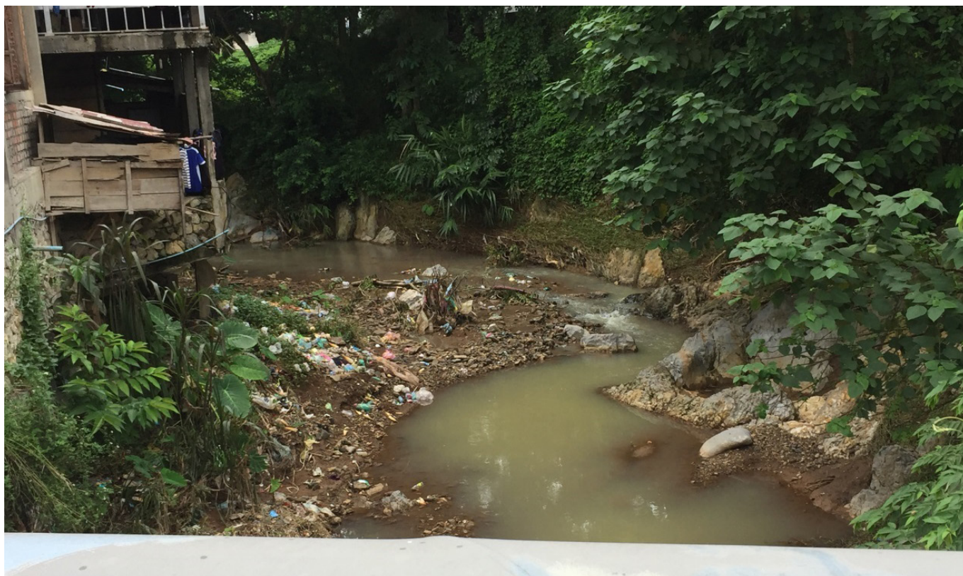
Site visit to a flood-prone area, near Luang Prabang, Laos. The siltation from upstream makes downstream situation worse each time. Houses around that area are adding additional floors to cope during the flooding periods as the first floors are often immersed in water for days and weeks.
