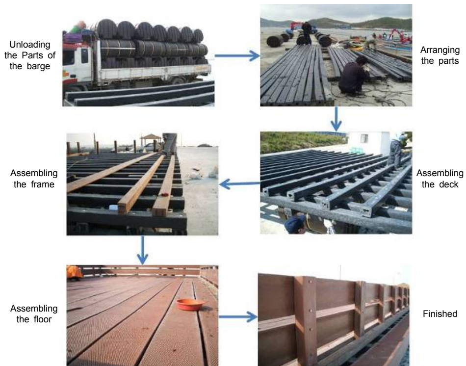
Figure 3. Process of building a floating receptacle for marine litter.
