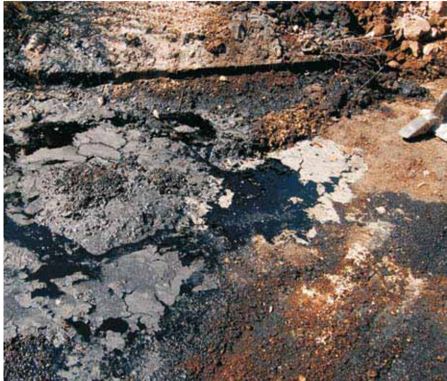
A pool of diesel and asphalt in the vicinity of the damaged tanks
