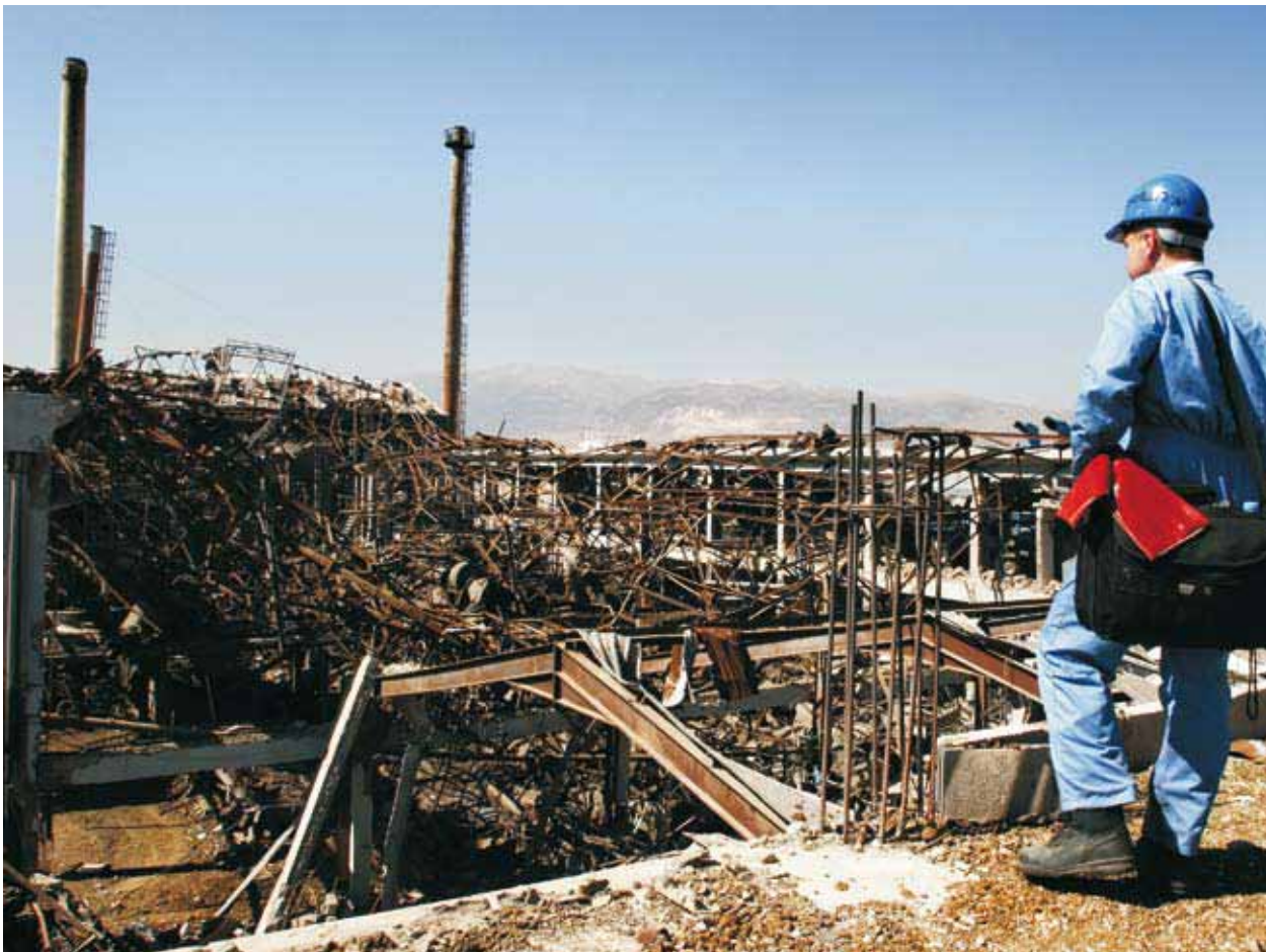
A view of the destroyed glass factory, with remaining chimney stacks in the background
