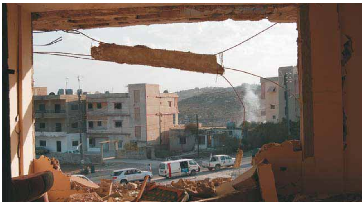
Site of the former Hannawiyah supermarket
