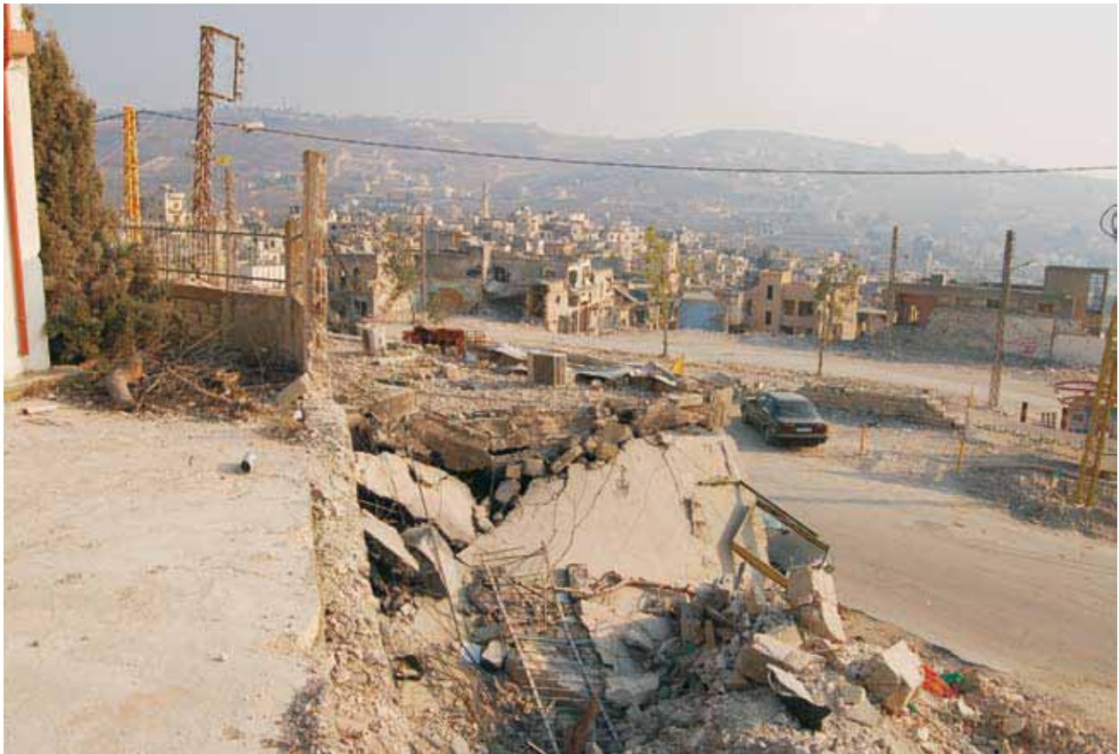
Site of a damaged school in Bint Jbeil, southern Lebanon
