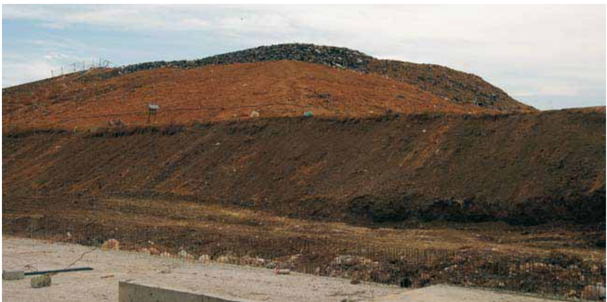
The Zahleh sanitary landfill, where good use of cover material minimizes problems with odours and pests
