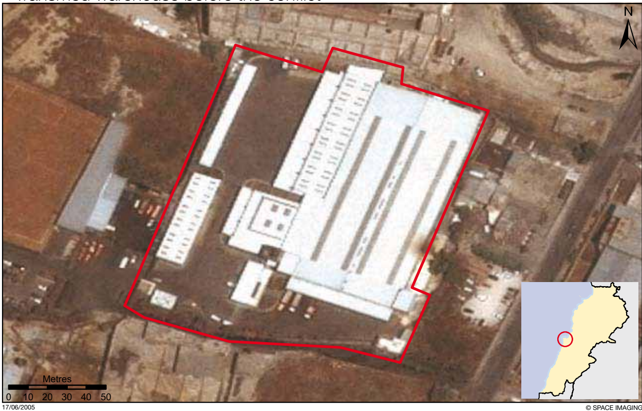
Transmed warehouse before the conflict
