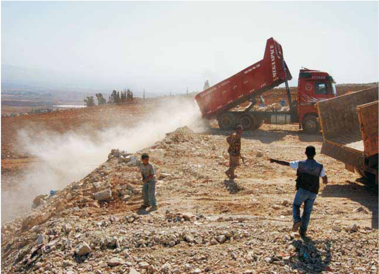
The Kham dump site illustrates the high levels of dust generation at most rubble disposal sites
