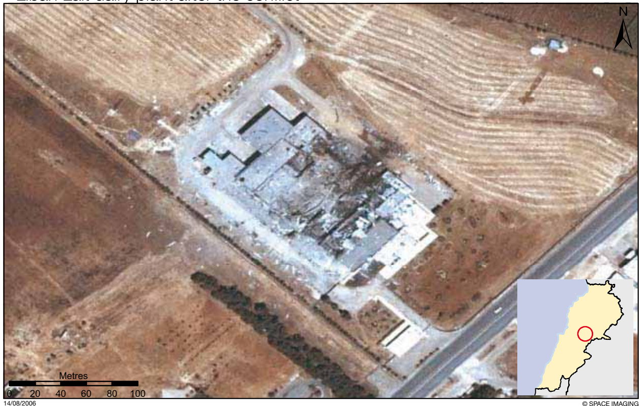
Liban Lait dairy plant after the conflict
