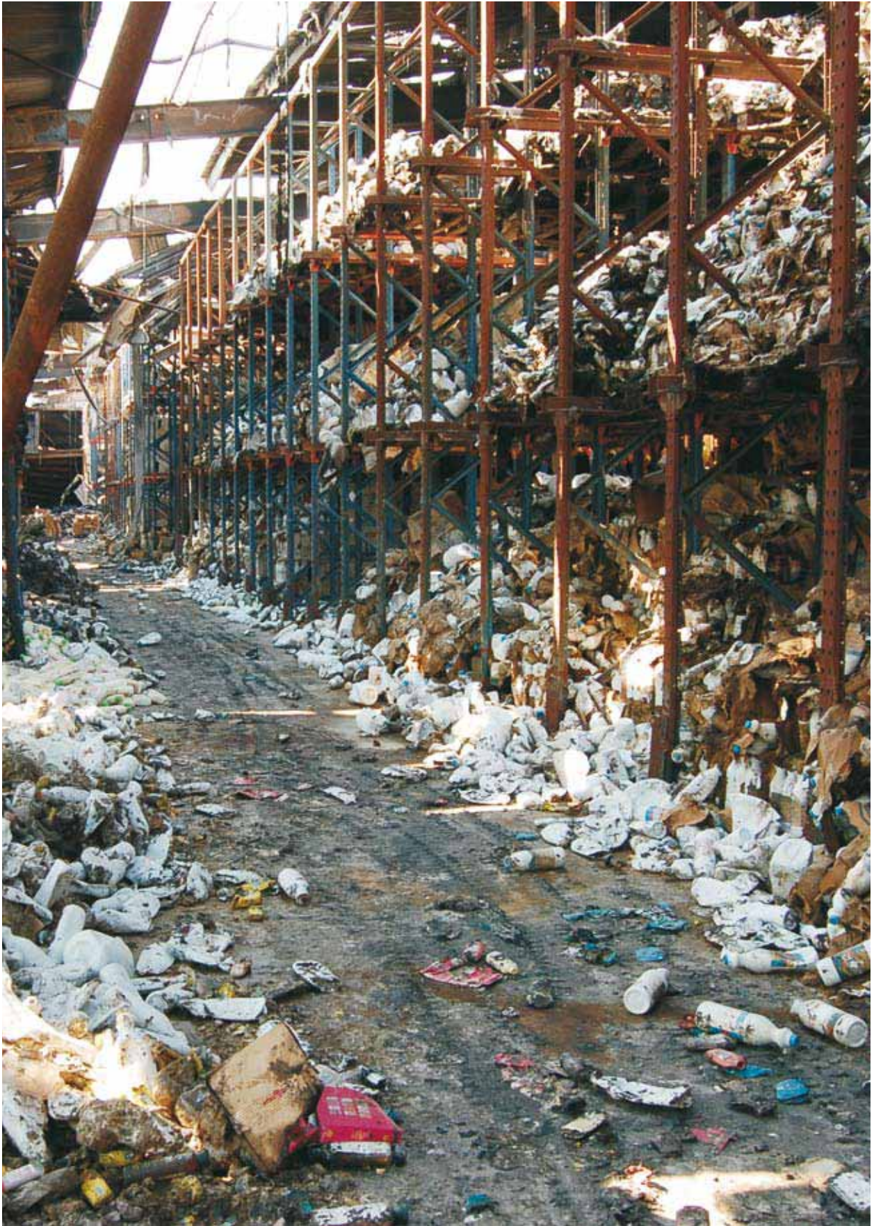
The interior of the damaged Transmed facility
