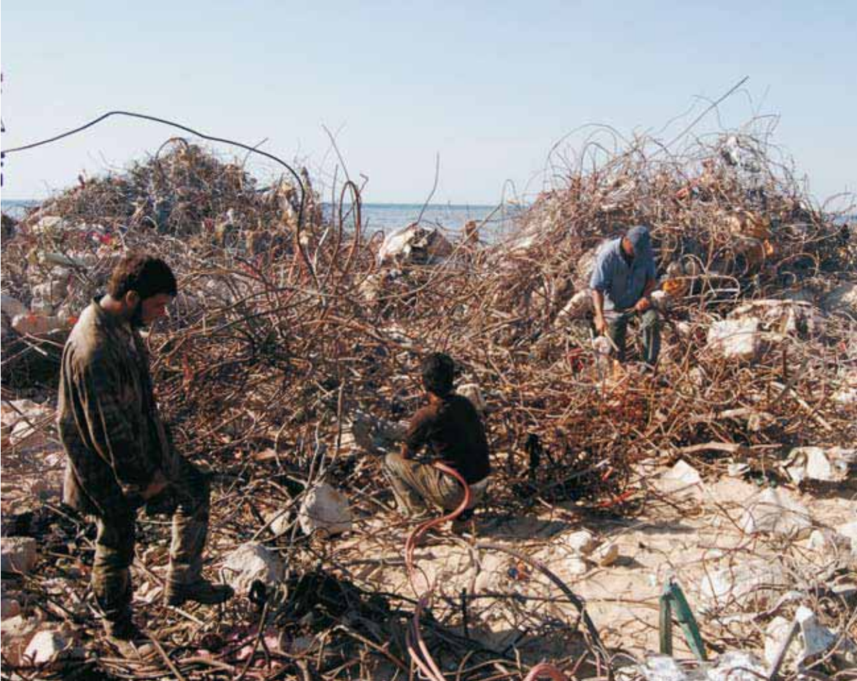
The lack of basic health and safety equipment, as seen here at the Ouzaii dump site, is a serious concern
