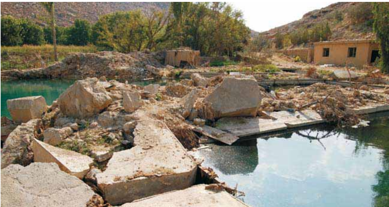
A view of the destroyed Al Maalaka fish farm
