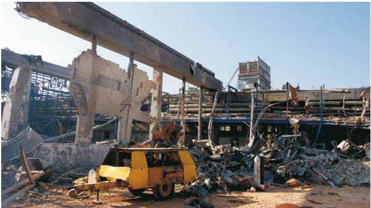
A view of the destroyed Liban Lait dairy complex
