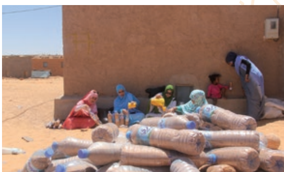
Women filling in plastic bottles with sand to use them as construction bricks. Credit Ecosahara and www.theswitchers.eu
