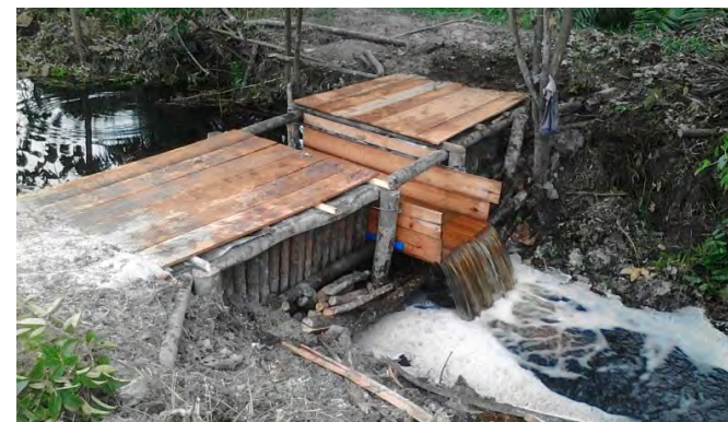
Figure 16. Canal Blockage for Rewetting Peatland
