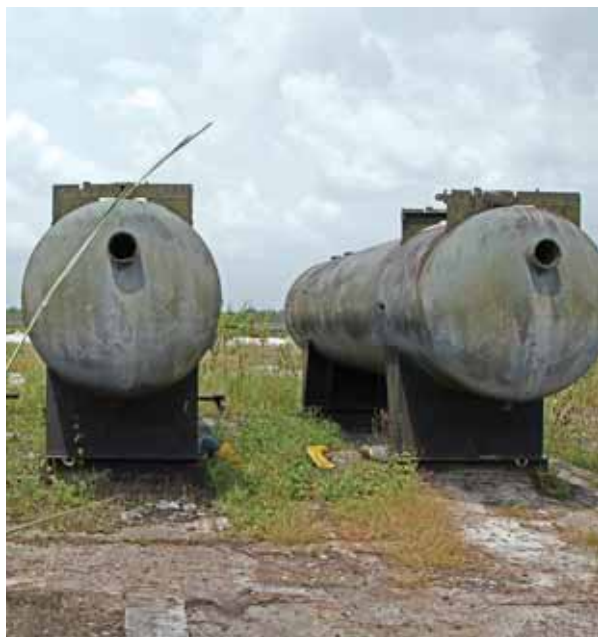
Abandoned oil field infrastructure (Bodo West, Bonny LGA)
