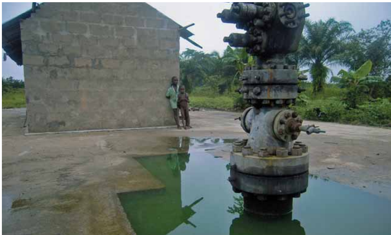
A house constructed on a well pad (Yorla 9, Khana LGA)
