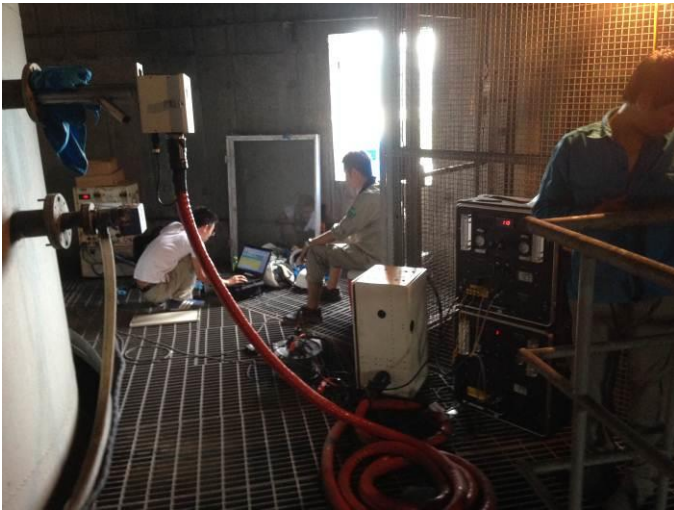
Hg and PM monitoring in Quang Ninh Thermal Power Plant
