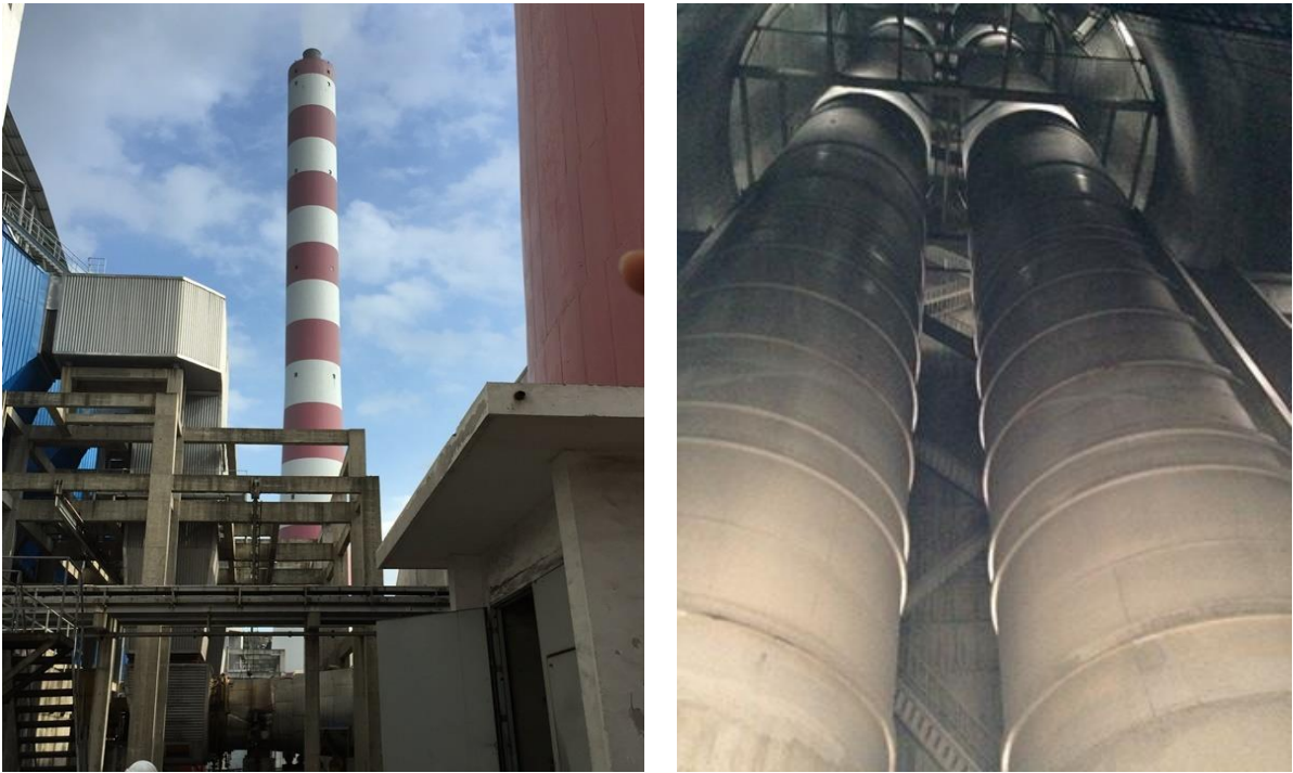
Figure 15. Stack of Quang Ninh coal-fired power plant
