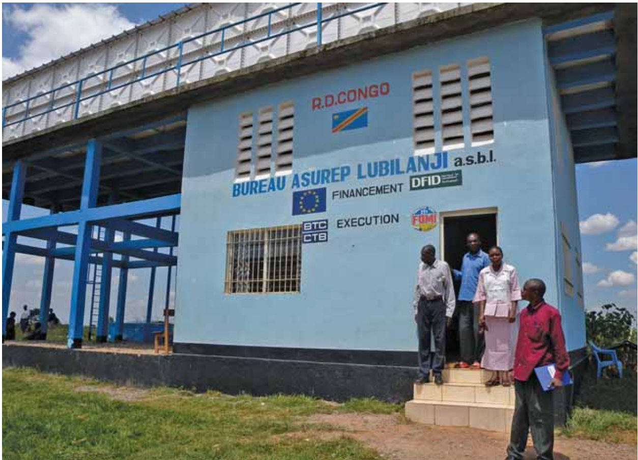
Newly constructed office of the Lubilanji Water User Association in Mbuji-Mayi, Kasai Orientale
