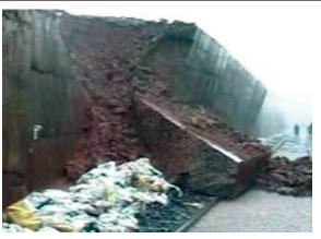
The collapse of retaining wall between Nivasar and Ratnagiri stations in Konkan Railway
