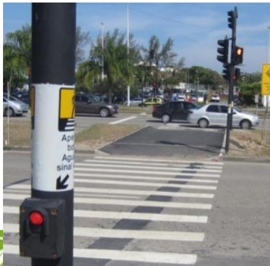
Signalized pedestrian crossing
