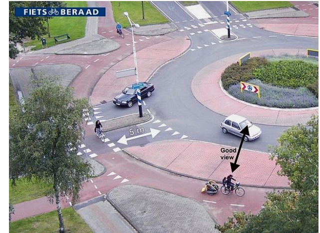
Roundabout treatment for bicycles, Enschede, Netherlands
