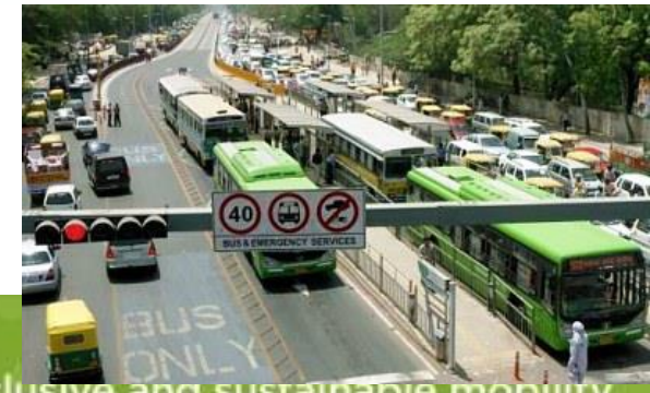
Bus lane in congested area
