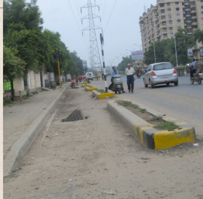
The revised road boundary being marked out adjacent to the ISRO wall on the Jodhpur Ramdevnagar stretch
