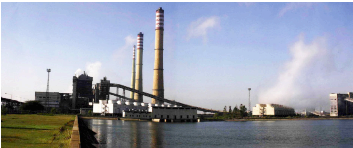
Figure 1 Suratgarh super thermal power station
