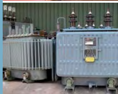
Dismantling of a PCB transformer
