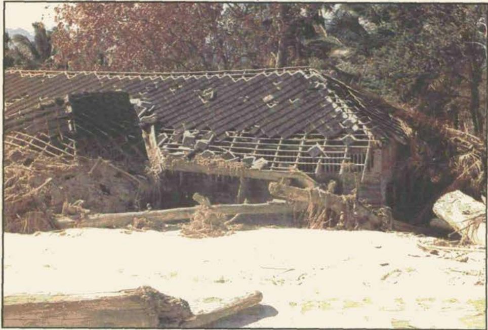
Fig. 14. The flood destroyed the houses.
