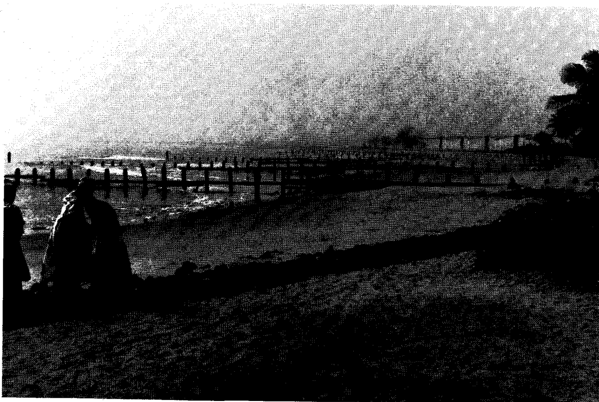
Fig. 5.3. - Beach protection at Cape St. Mary (Gambia) by using wooden groins. (Quélenec, 1988).
