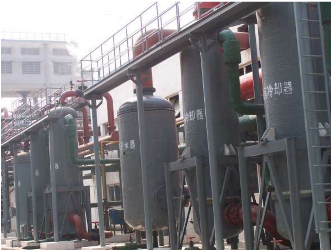
Figure 4-1 A vinyl chloride monomer (VCM) production plant in China
