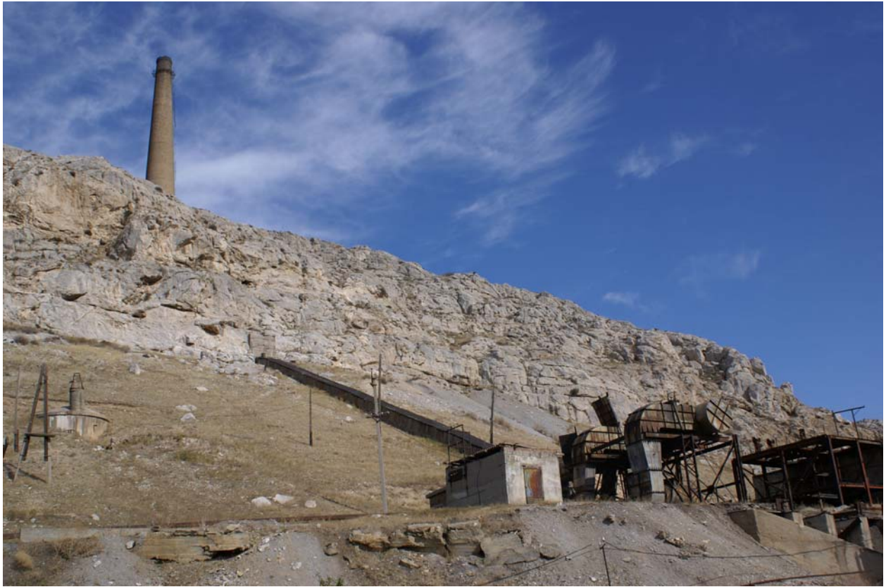
Figure 19 Mercury smelter stack
