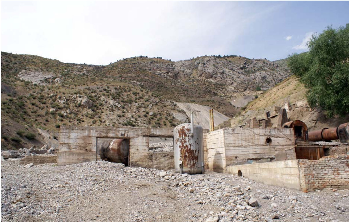
Figure 31 Chauvay mine: Dismantled rotary kilns and smelter. July 2008
