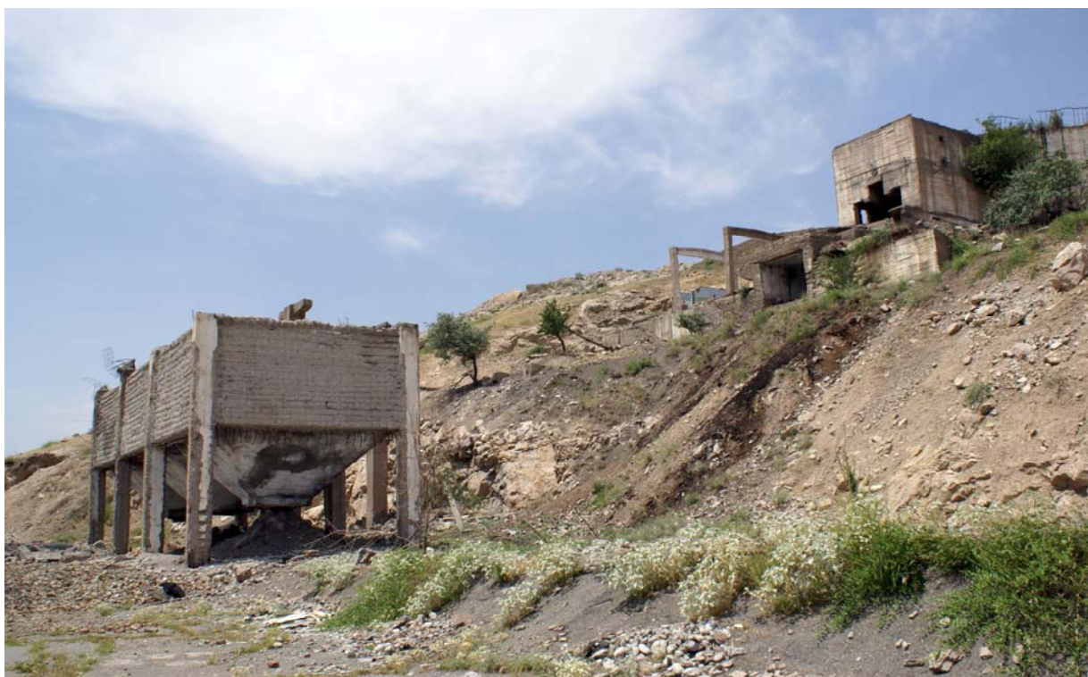
Figure 30 Chonkoy-Ulug-Too mine: Dismantled ore milling section. July 2008
