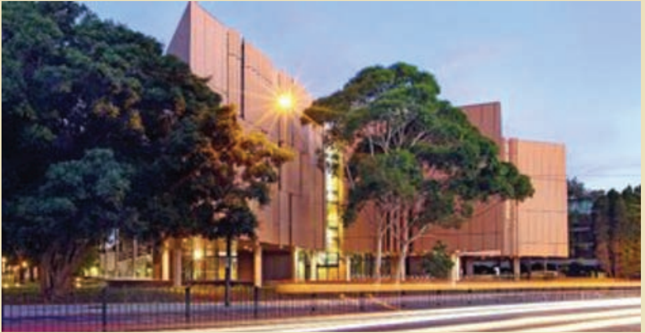
Tyree Energy Technologies Building (TETB), University Of New South Wales (UNSW)
