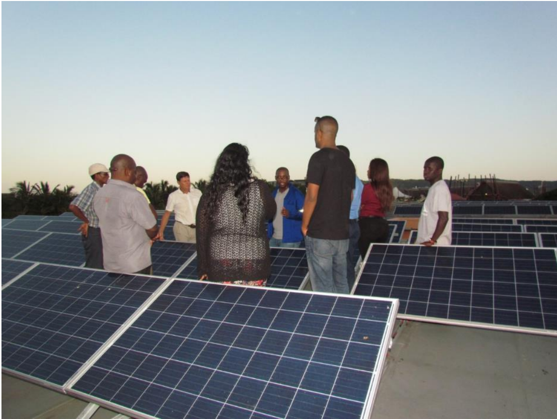
Figure 12: Solar panels installed on the rooftop at Ushaka Marine World.
